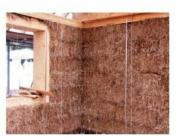
Figure 8: A completed wall with straps connecting the wall plate to the base
