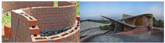
Figure 6: Rat-trap bond for curved wall
